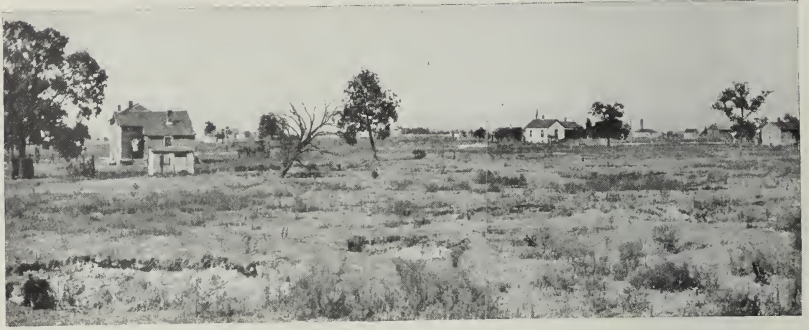
FIG. 18.—Large area covered by pit holes in the suburbs of a town in central Illinois where a 5-foot bed of coal is being mined at a depth of 75 to 100 feet. Trees are falling into the pit holes; the houses are being used.
